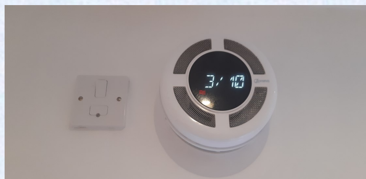
A small MVHR extractor fan suitable for one room.
