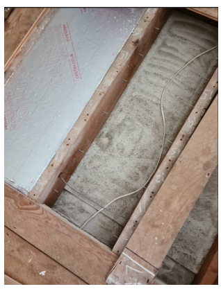
Lifted lounge floorboards to install insulation
