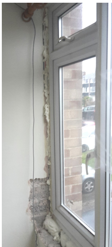
Expanding foam fills gaps
